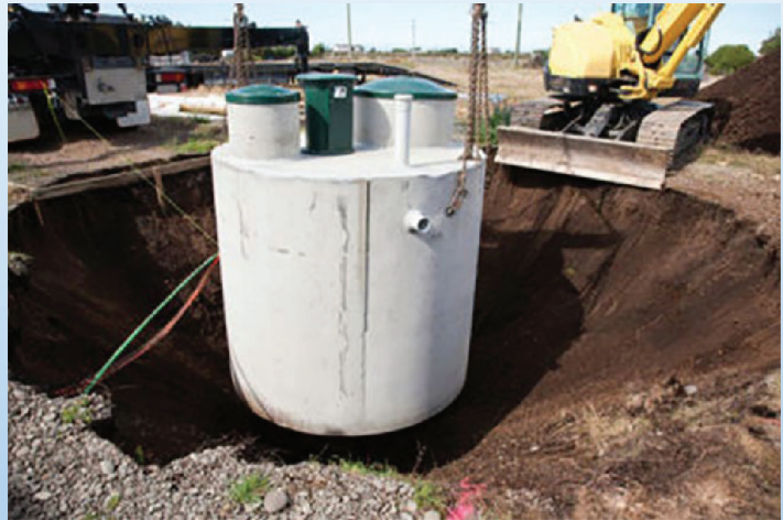
An ATU pumps oxygen to accelerate the natural process of breaking down organic material.
