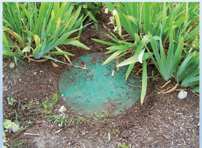
Orencia 1,500-gallon tank and block-lined seepage pit
