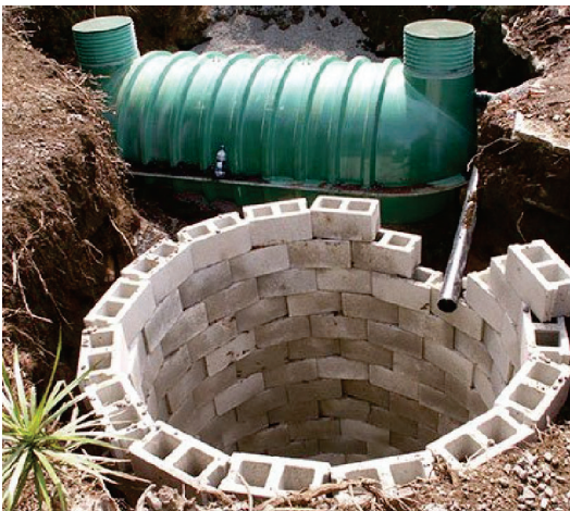
Orencia 1,500-gallon tank and block-lined seepage pit
