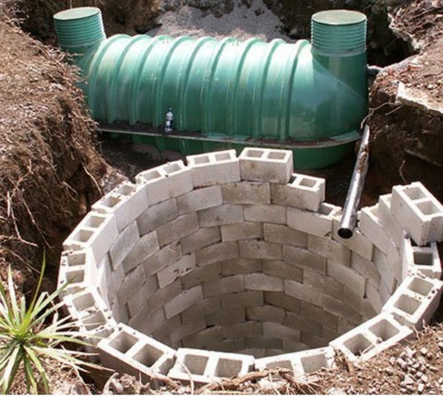
Orencia 1,500-gallon tank and block-lined seepage pit
