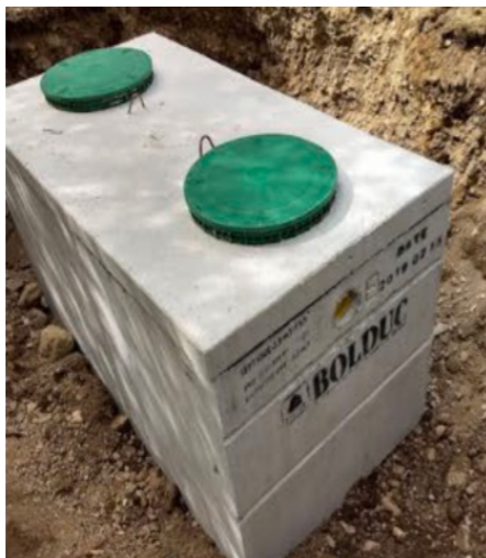
Rectangular, Concrete Tank
