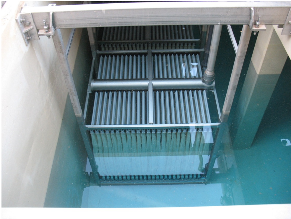
Figure 5-8. Membrane Cassettes at Johns Creek Environmental Campus, Fulton County, GA
