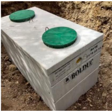
Rectangular, Concrete Tank
