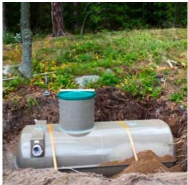
Steel, Horizontal, Cylindrical Tank
