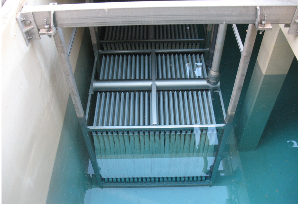
Figure 5-9. Membrane Cassettes at Johns Creek Environmental Campus Fulton County, Georgia
