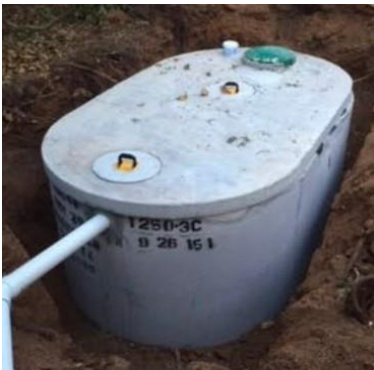
Oval, Concrete Tank
