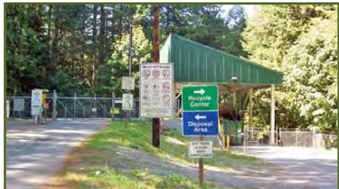
Automated Rural Drop Box Pay Station in Skykomish, WA Source: King County (2018)
